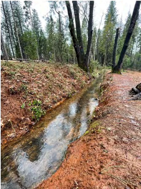
Image 8: Corner #4. Looking straight across to corner #5.
